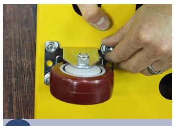
Install the casters using 4 bolts and nuts.
