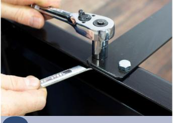
Fully tighten with a 1/2" wrench and socket.
