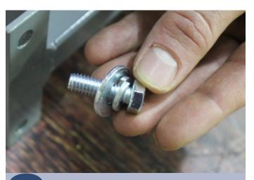
Attach using a 1" L 5/16" bolt with a lock washer and standard washer. Tighten down with a 1/2" socket. Repeat for all bolts on both sides.
