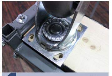
Align the caster over the provided holes. The swivel casters will go on the end with the handle. The rigid casters go on the opposite end.
