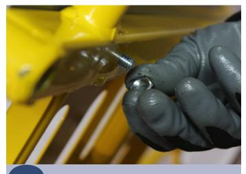
Finger tighten the lock nut onto the carriage bolt. Repeat steps 2 & 3.
